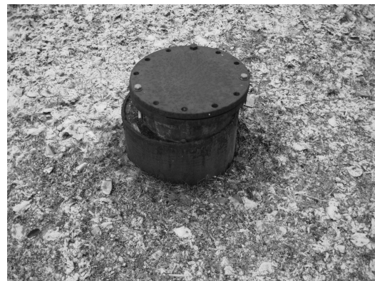
Figure 8.6: View of the F99 well head (February 2008).
