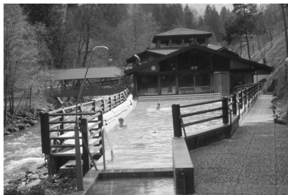
Figure 12.2: View of the Val d'Illiez spa (photo : H Rickenbacher, 1998)
